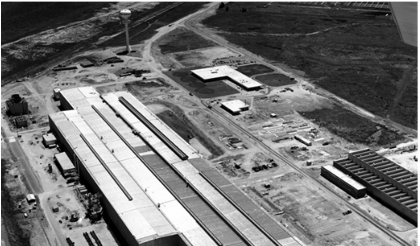
The Ensenada unit. It took 33 months from project design to the facilities' start-up.
